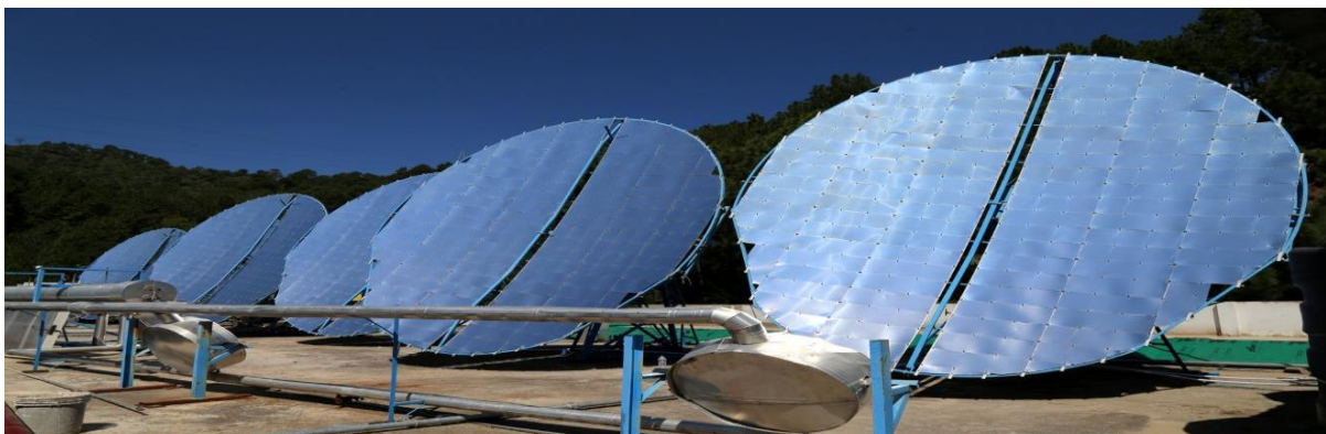
Concentrated Solar Power Steam Cooking System for 500 at Girls Hostel, Shoolini University, Solan, Himachal Pradesh
