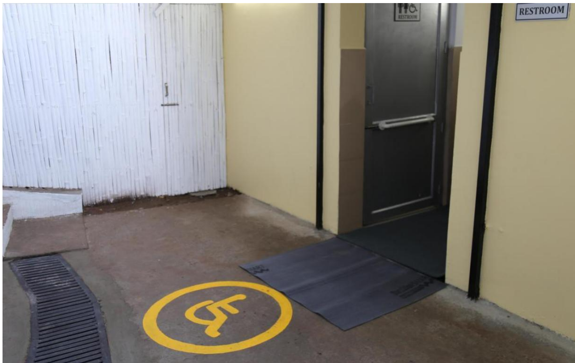
Washroom near Director Operations office
