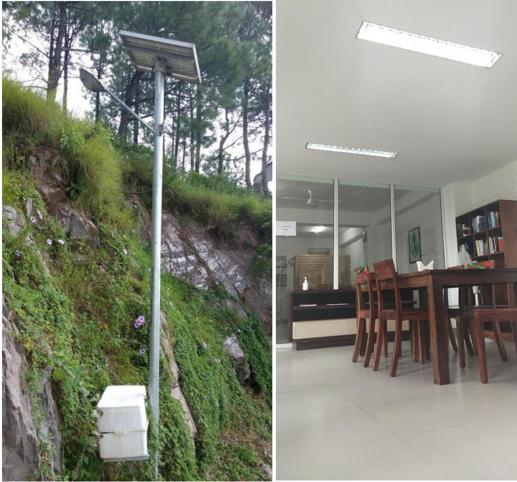
Figure 13: Utilizing clean Solar energy -Solar street lights installed in the university Campus(left) and use of energy efficient LED lights inside the university buildings (right)
