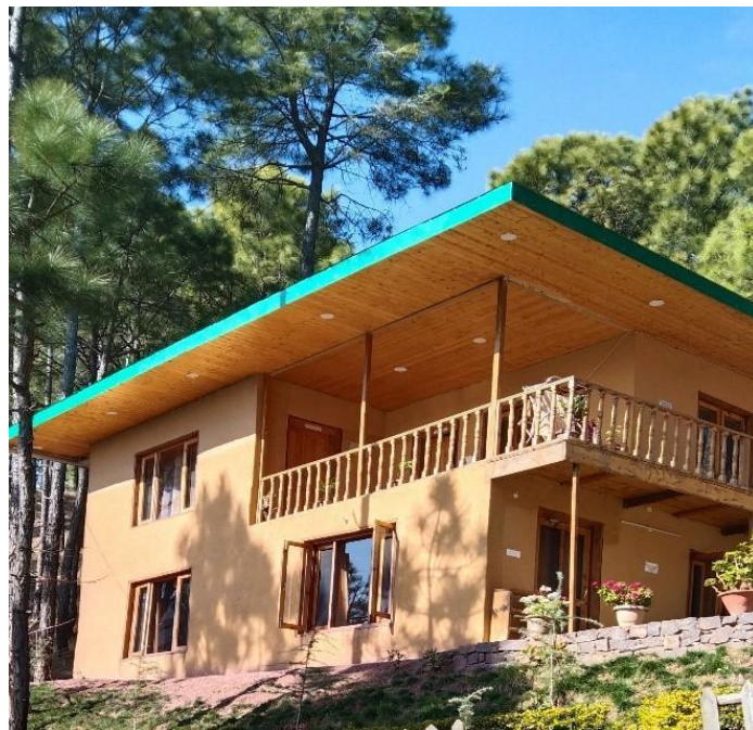
Figure 6: Sustainable building with mud walls in Yogananda Ville at Shoolini University.
