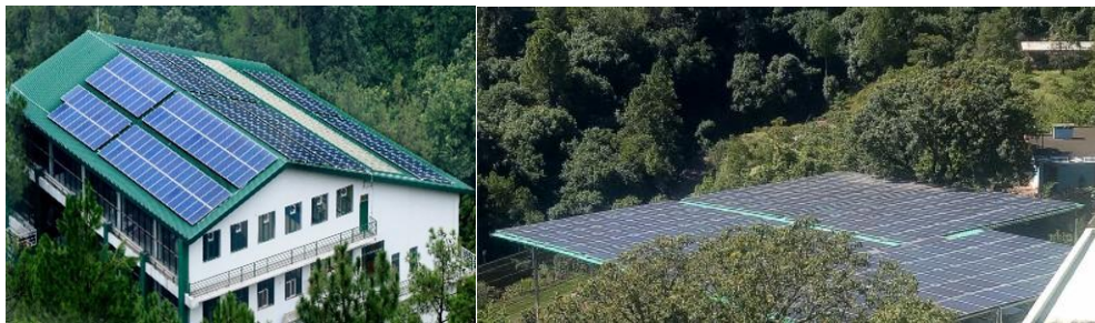
Figure 2: Distribution of 400kWp grid-connected Solar Photovoltaic Power Plant on different rooftops and Car parking shed in the university campus
