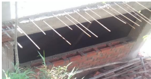
Figure 16: Walls with Rat traps for better insulation and thermal comfort
