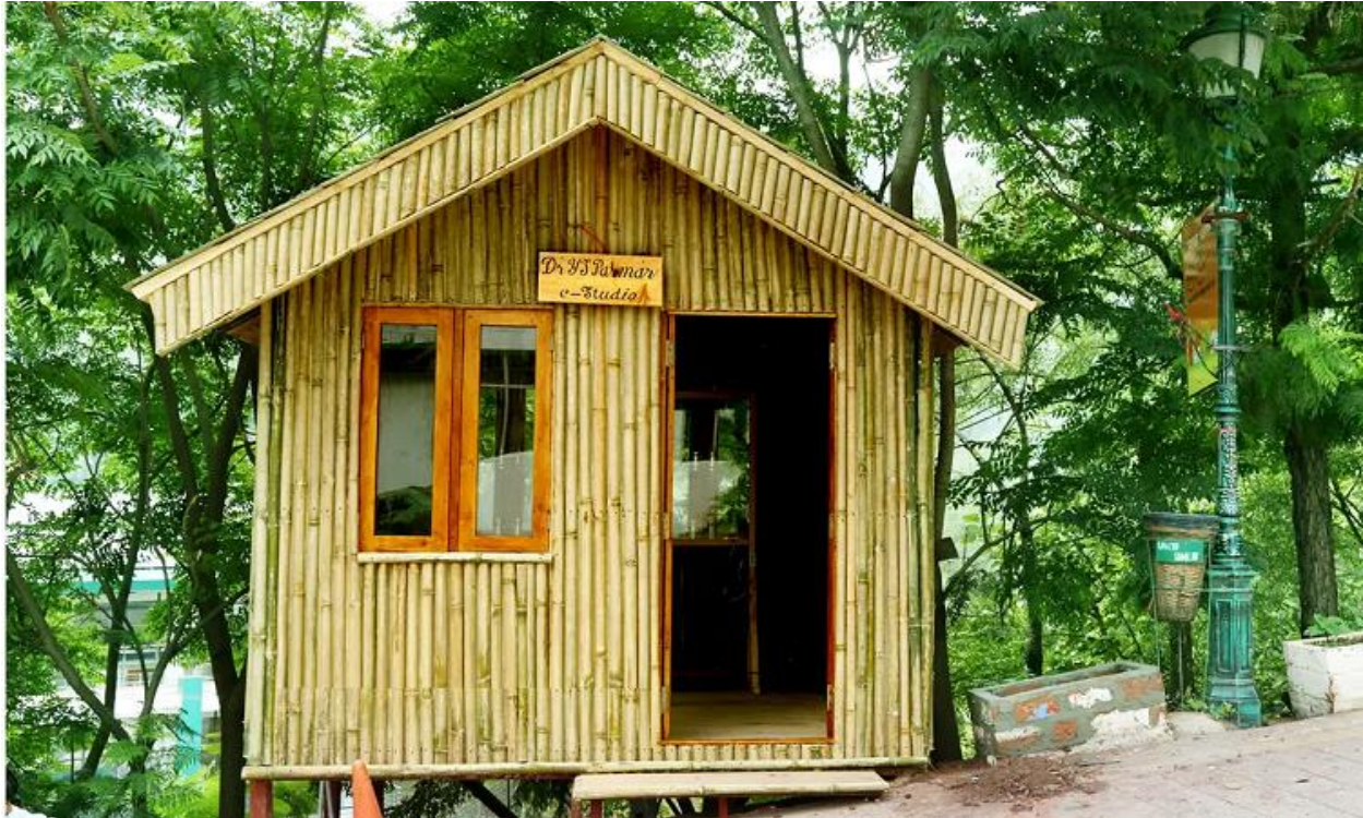
Figure 22: Bamboo and slate Roof E-Studio for online lectures constructed during COVID times
