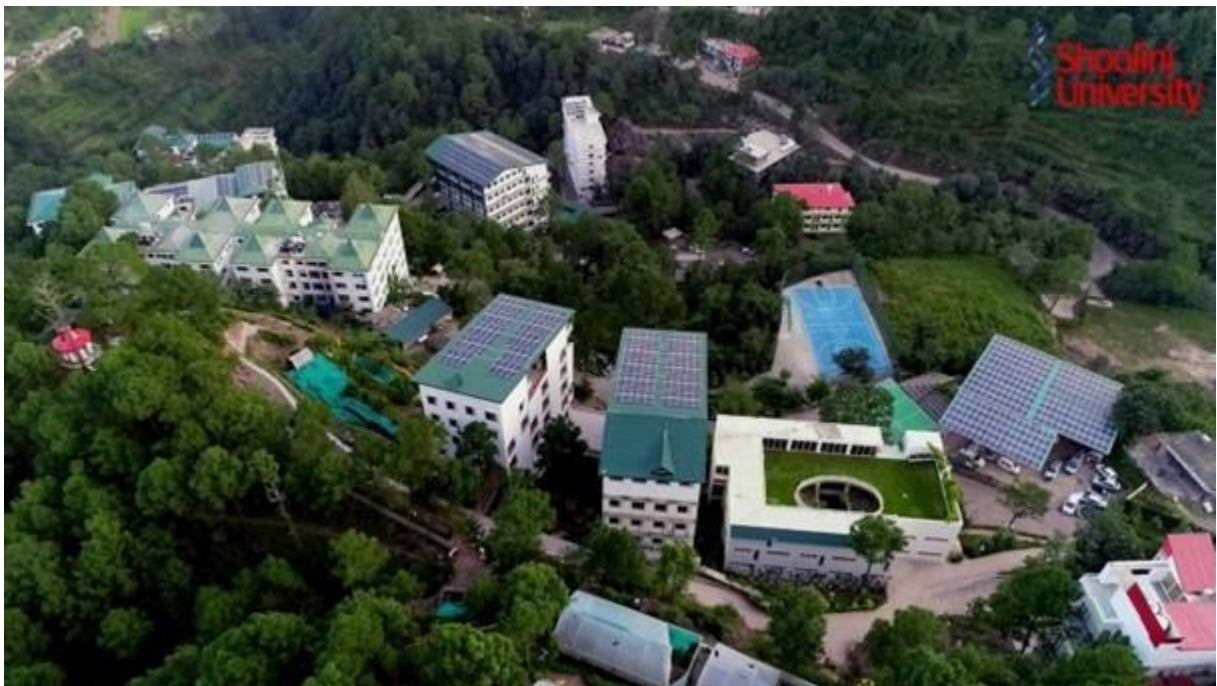
Figure 1: 400 kWp Grid connected Solar Photovoltaic Power Plant at Shoolini University
