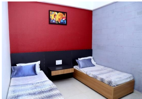
Figure 15: Walls using AAC blocks for better insulation and energy efficiency
