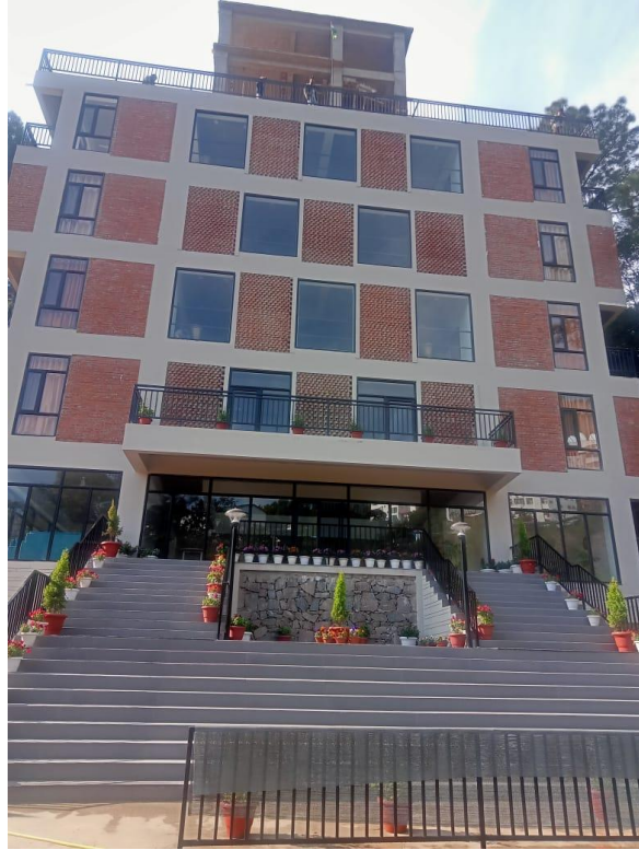
Figure 14: Use of large windows for increased solar gain and increased use of natural lighting.
