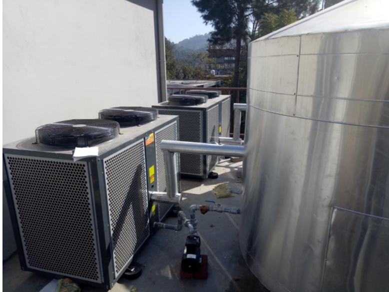
Figure 12: Energy efficient heat-pump based water heating system has been installed in the international hostel Shoolini University
