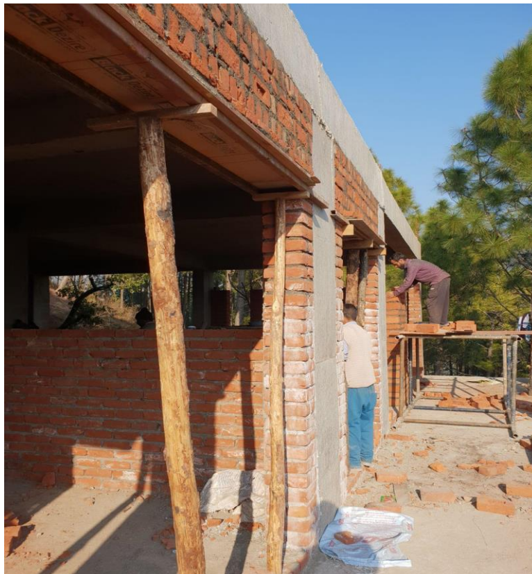
Figure 9: Walls with Rat traps for better insulation and thermal comfort
