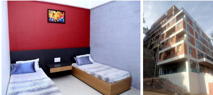
Figure 10: Walls using AAC blocks for better insulation and energy efficiency
