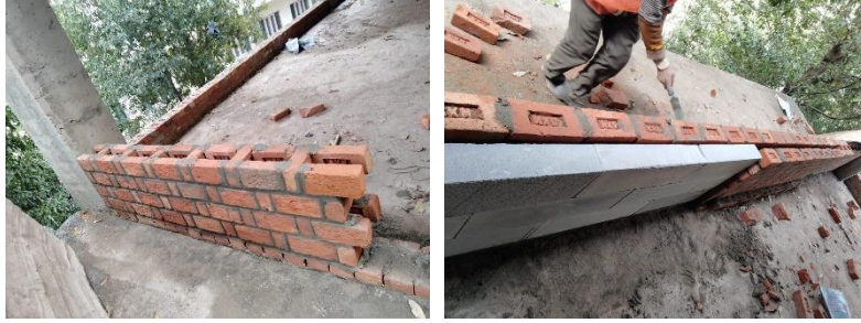
Figure 1: Training to Masons in Air gap brick walls and composite block walls being used for improving insulation and thermal comfort.
