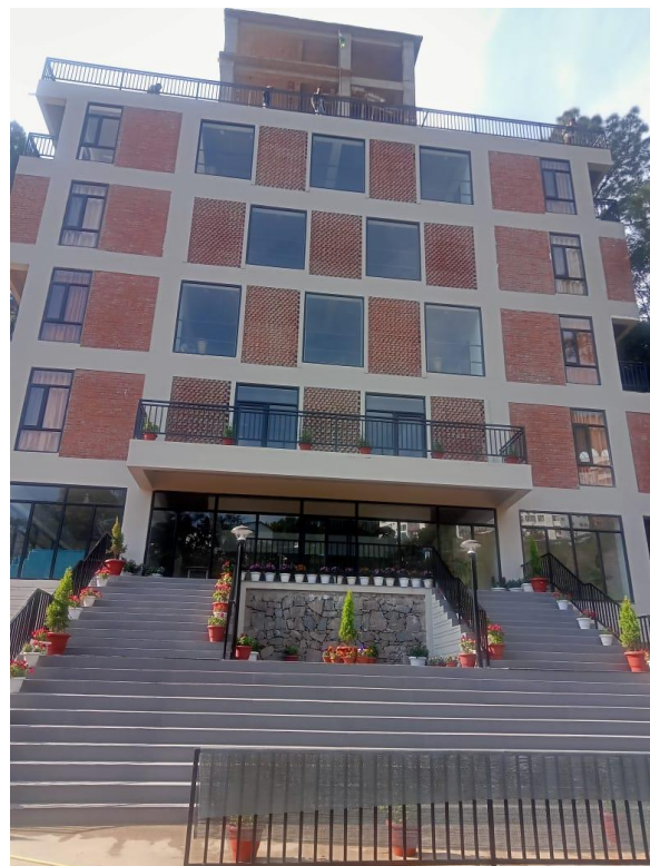
Figure 11: Use of large windows for increased solar gain and increased use of natural lighting.
