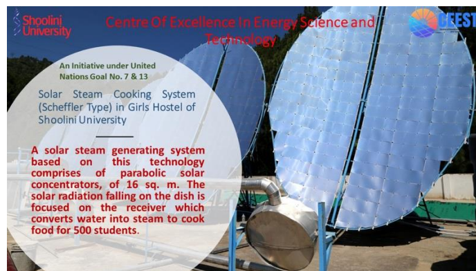
Figure 3: Steam cooking system for 500 students at girls hostel rooftop at Shoolini University
