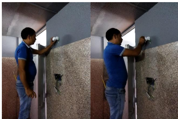
Energy efficient device installation
